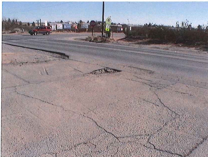
Figure 20 - Chaparral ES Main Parking Exit
