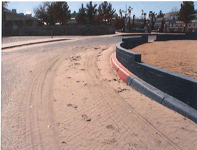
Figure 9 - Sunland Park ES Main Circle Drive
