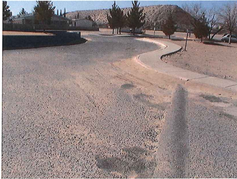
Figure 8 - Sunland Park ES Main Circle Drive
